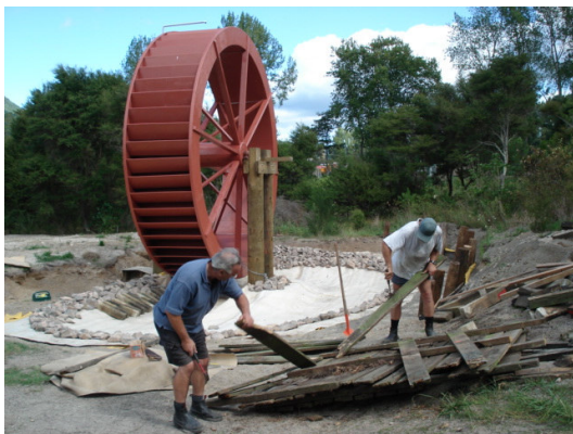
Work being done on the pond by trust members for the full scale replica water wheel built by Stan Fretwell.
